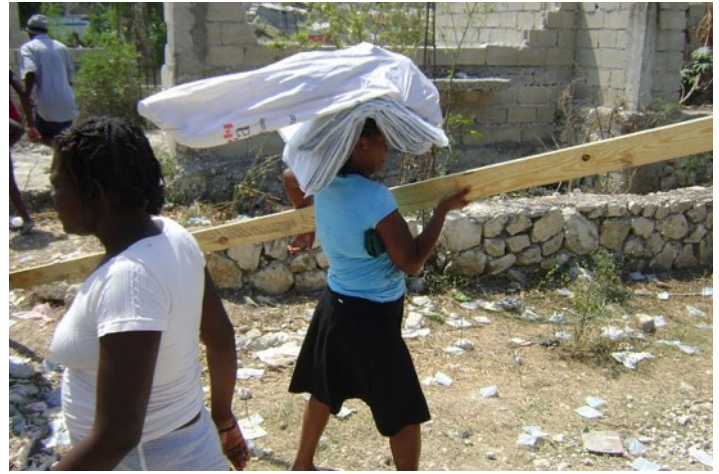
Each family received materials for building a shelter, including two tarps, a 12' beam, saw and shovel.
