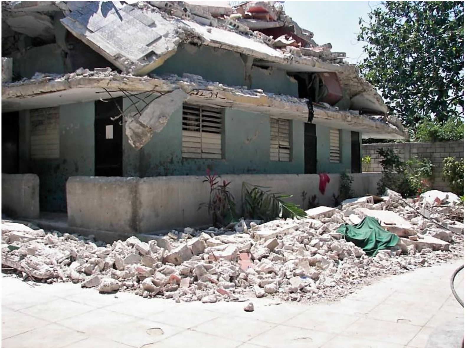
This orphanage building in Léogâne collapsed during the earthquake. Two people were killed and one girl lost both her legs.
