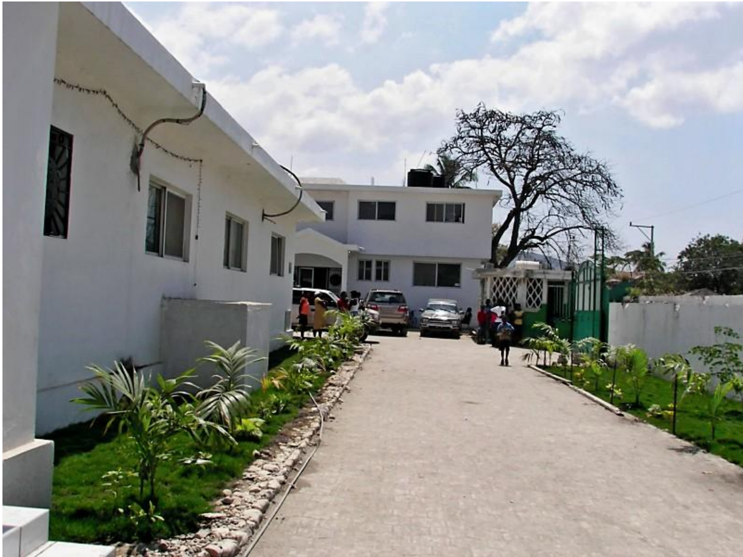
The hospital of St. Marc is an example of successful partnership between the Government of Haiti and Zanmi Lasante. This well-equipped hospital now receives running water through a public system funded by the Inter-American Development Bank.
