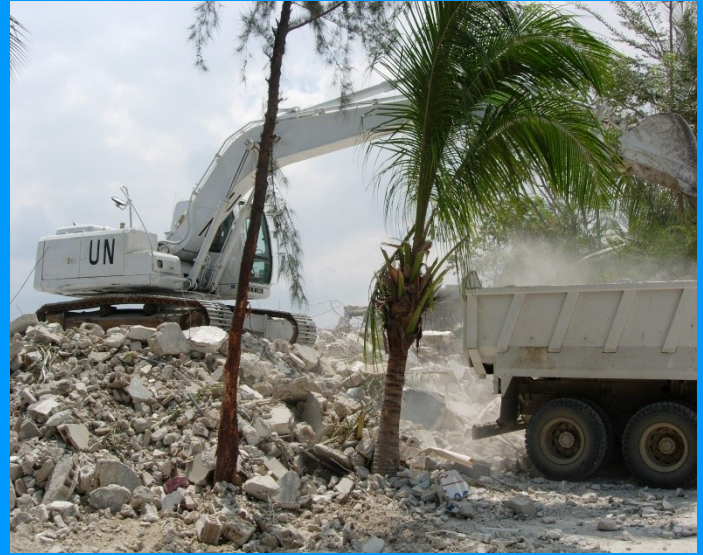
MINUSTAH forces begin rubble clearance at a local primary school.
