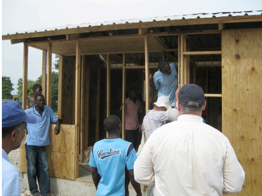
Fig. 6: “T-shelters,” semi-permanent transitional shelters, are being constructed at many relocation sites, including at the Tabarre Issa Emergency Relocation Camp. While durable, the T-shelters have been more expensive than budgeted, and their construction has been delayed due to supplies being held up by Haitian Customs officials. It has been estimated that 125,000 T-shelters have been donated (which could house up to 600,000 people), but the land upon which to build and place them has yet to be identified by the Government of Haiti. June 8, 2010
