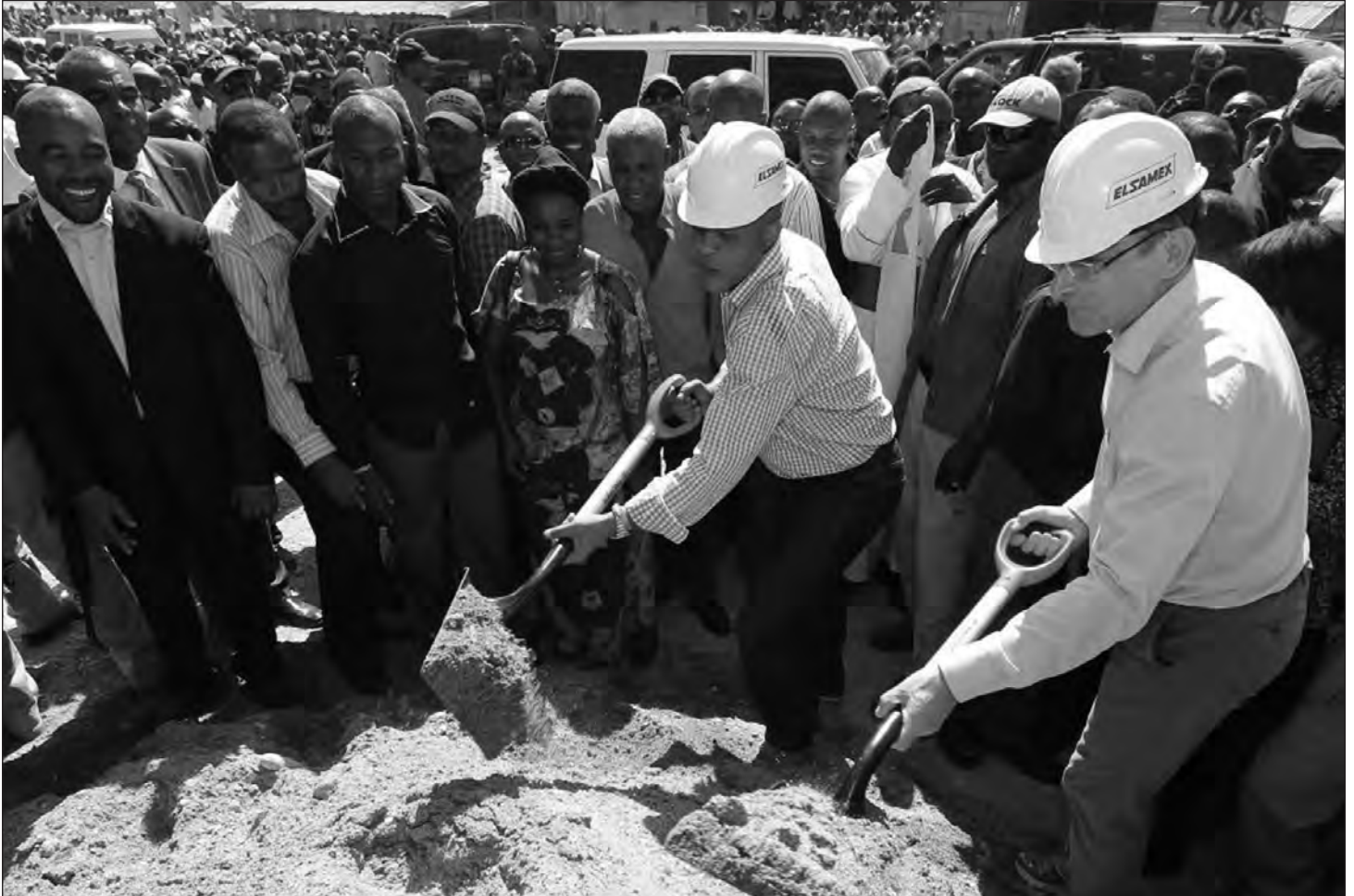
Shovel-ready for poverty eradication or just building roads? President Michel Martelly poses with EU Development Commissioner Andris Piebalgs to start work on the third leg of the EU-funded National Route 3 from Hinche to Cap Haitien. Source: Michel Martelly Facebook page
